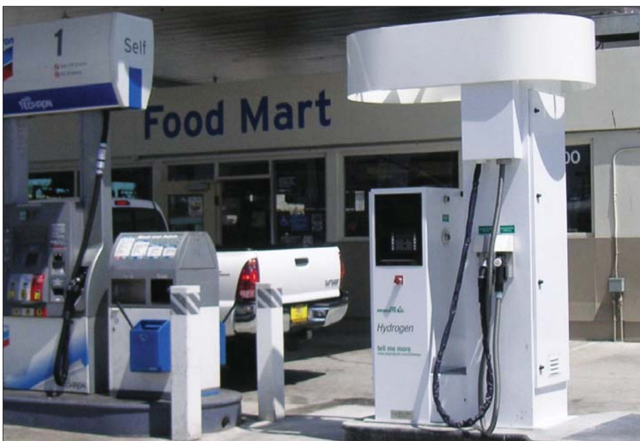
Air Products' hydrogen fuel dispensing technology placed at this retail gasoline station in California, part of a step change in infrastructure capabilities, is part of a "compression-less hydrogen fueling station."
